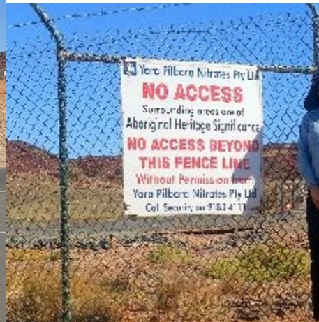
Condition 8: 2.5 m chain link perimeter fence and signage near main entrance/exit
