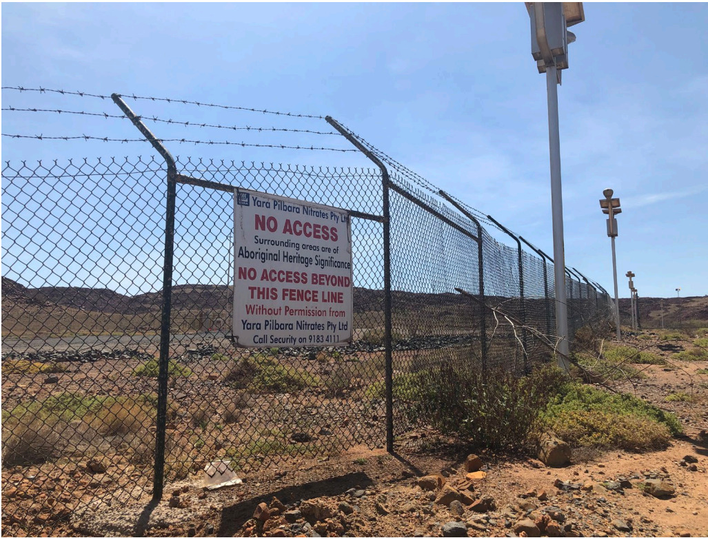
Condition 8: 2.5 m chain link perimeter fence and signage near Integration Road entrance/exit
