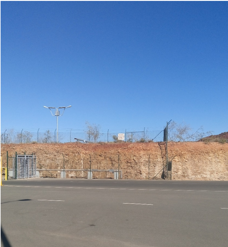
Condition 8: 2.5 m chain link perimeter fence and signage near main entrance/exit
