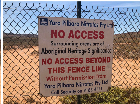
Condition 8: 2.5 m chain link perimeter fence and signage near emergency exit
