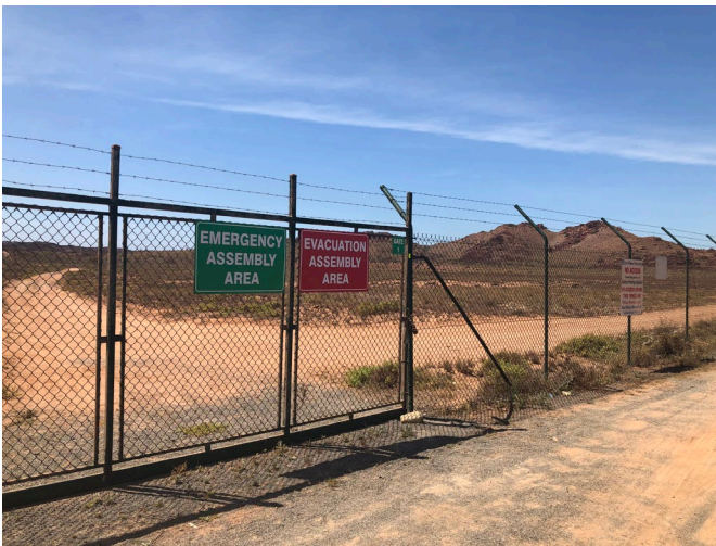
Condition 8: 2.5 m chain link perimeter fence and signage near emergency exit
