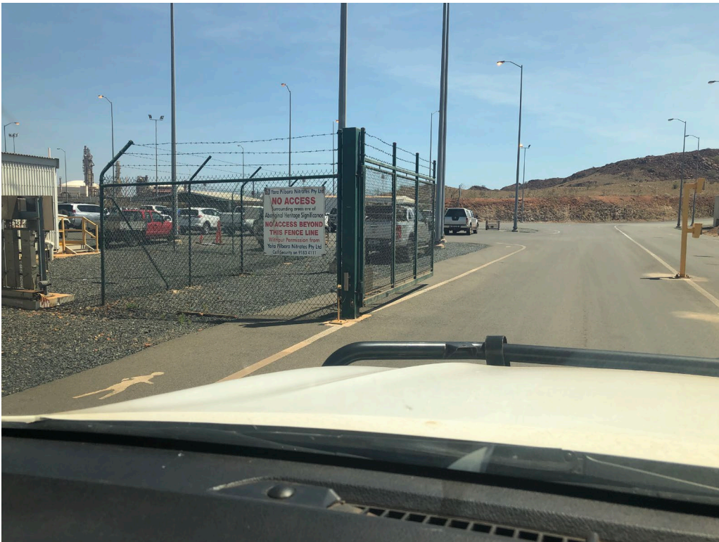
Condition 8: 2.5 m chain link perimeter fence and signage near truck parking entrance/exit
