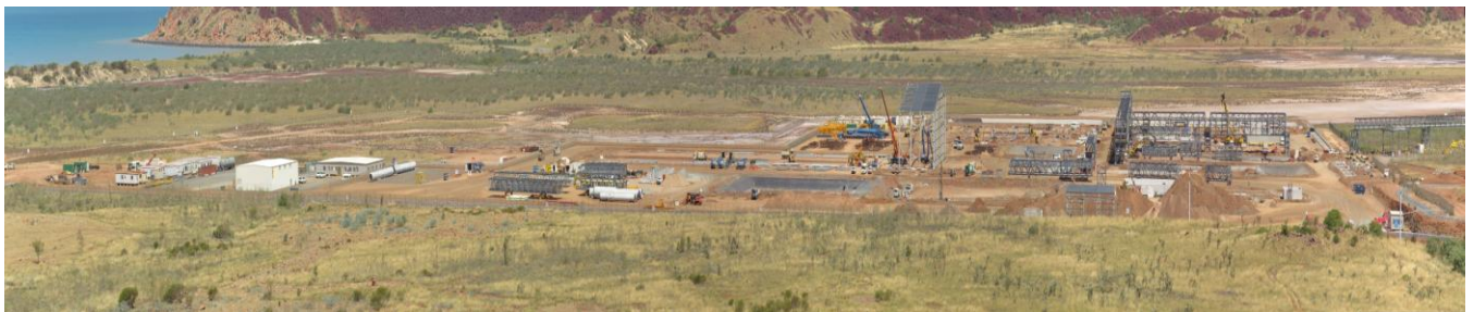
Figure 4: Technical Ammonium Nitrate Production Facility (TANPF) (March 2014).
