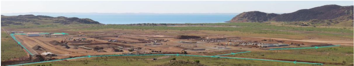
Figure 13. North West Creek diversion.
