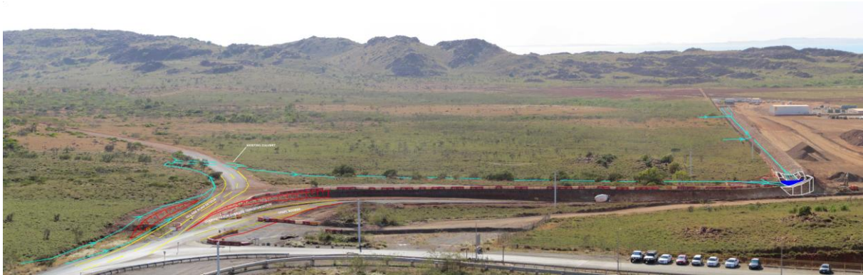
Figure 14. North Creek diversion once complete.
